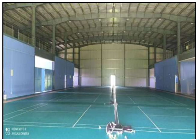
Fig-6: Multipurpose Indoor sports Hall Dibrugarh
